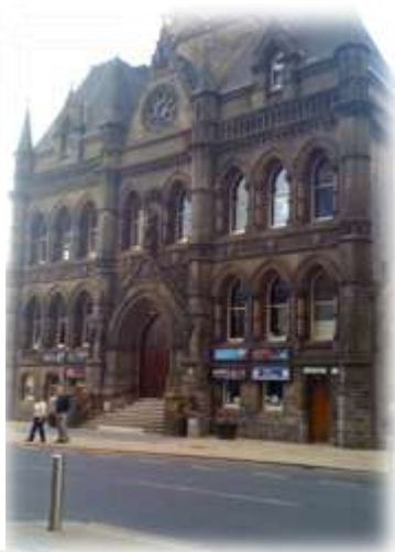
Venue: Middlesbrough town hall
